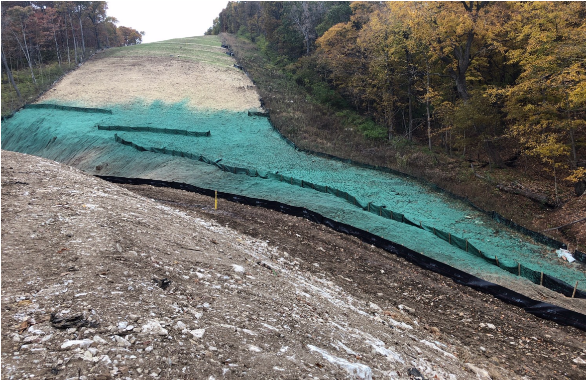
MP 45.0 capturing final ECDs and final hydro mulching. The photo was captured facing north.
