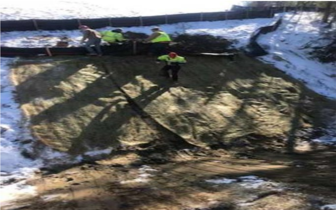
PAR #56 where Spire recontoured the slipped stream bank of stream SIL-JJP-130. The disturbed area was seeded and curlex was added for stabilization. Photo was captured facing south.
