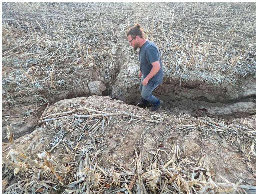
Photo 3. 3 - 4 Feet Deep Erosion Gully Over Operating Pipeline
